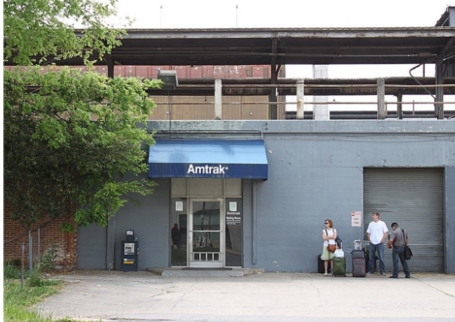
Access to the current Birmingham station is through this street-level entrance. Photo by Ralcon Wagner
